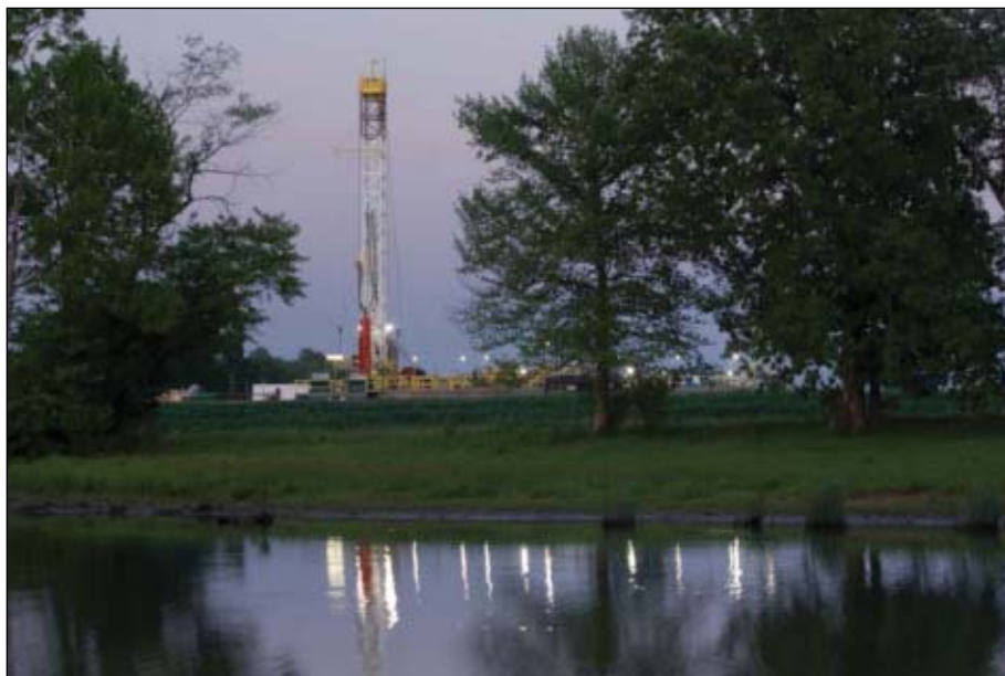
DeSoto Drilling Inc. has 10 Cowan MD-500 super single rigs drilling the Fayetteville shale for Southwestern Energy. This rig was drilling in 2007 (Fig. 2, photo from Southwestern Energy Co.).
